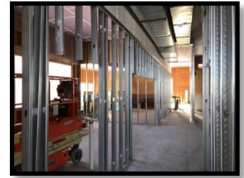
Walls being framed and duct work being hung.
