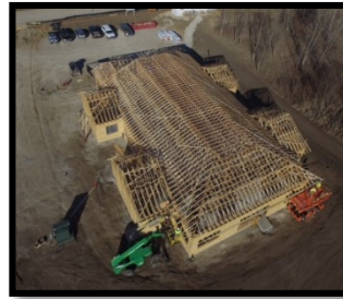
Arial view of the new hospital before sheeting and roofing.
